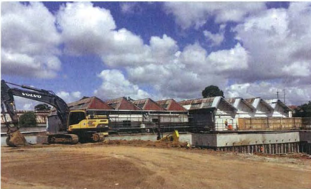
Figure 6. Ongoing construction at 20 Shepherd Street Source: Mecone
