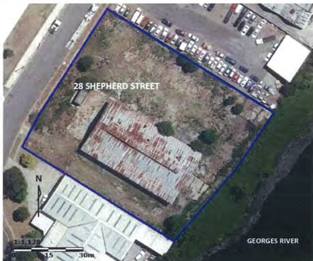
Figure 9 - Site location at 28 Shepherd Street, Liverpool, an abandoned warehouse facility, the eastern boundary contiguous with vegetation along a section of the western embankment of the Georges River
